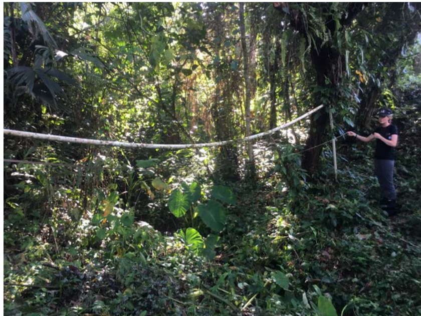
Figure 8. Existing Pipe Bridge (Photo by: Hailey Goupille)
