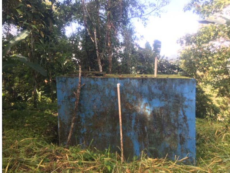
Figure 7. Existing Holding Tank Provided from the Panamanian Ministry of Health (Photo by: Hailey Goupille)
