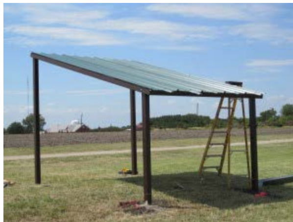
Figure 14. Sample Rainwater Catchment Roof [3]
