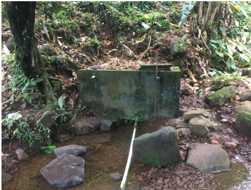
Figure 6. Existing Spring Box Provided from the Panamanian Ministry of Health (Photo by: Hailey Goupille)
